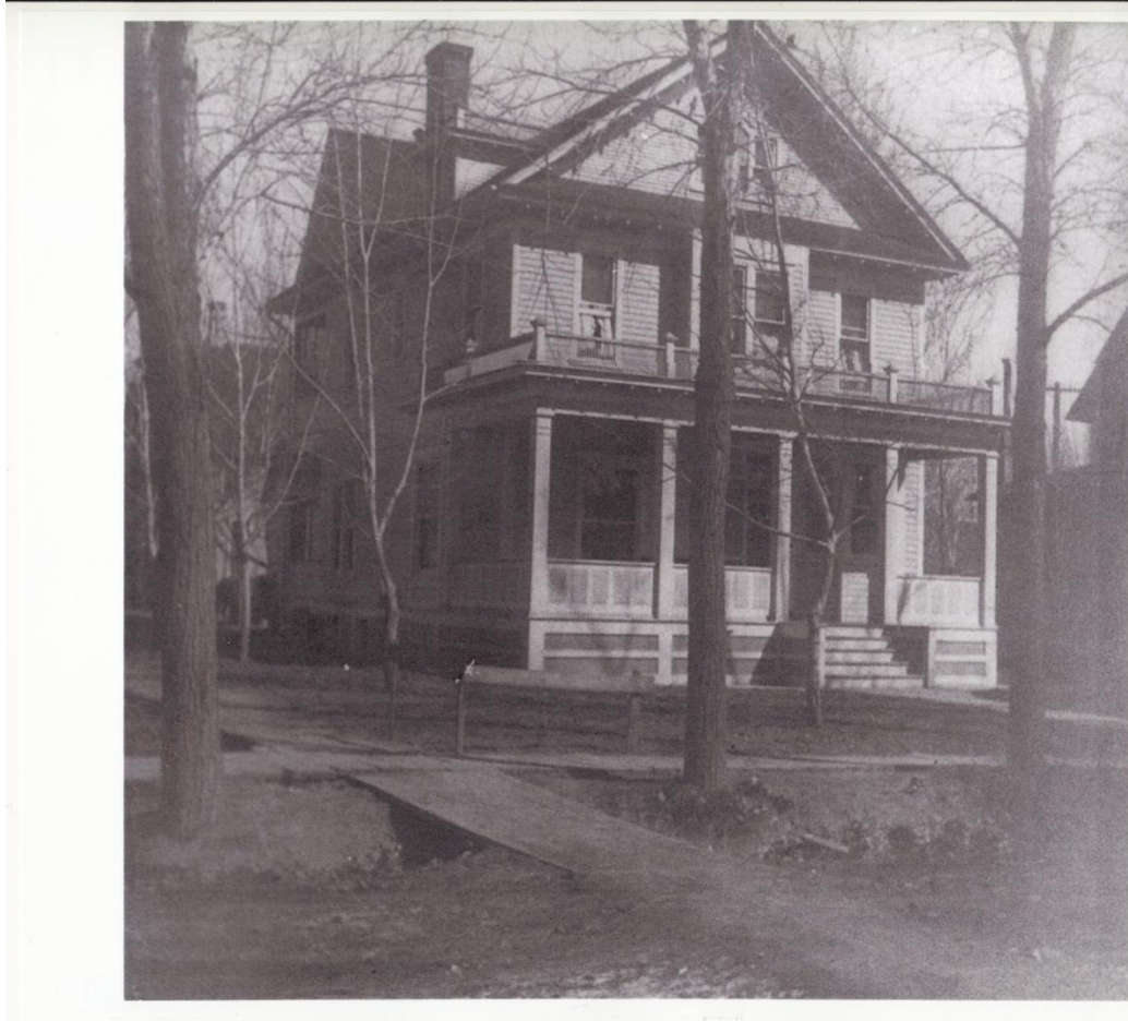
The irrigation ditch running in front of 440 N. Seventh Street supplied the water for the trees planted in front of the house. The photo shows a small pipe going from the ditch that supplied water to the tree in the middle. the trees to the right of the boardwalk remain today. Kathy Jordan photo collection.
