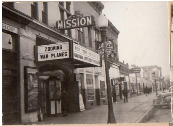
The Strand Theatre opened at 349 Main Street in 1928 and in 1935 it was renamed the Mission. In 1945 the named was changed to the Joy Theatre. Loyd Files Research Library Museum of Western Colorado photo file
