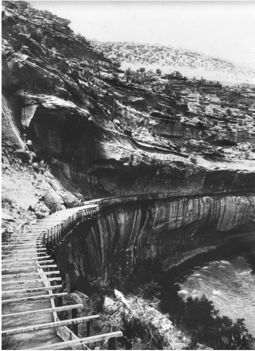
Hanging Flume, taken in 1891 shortly after it was completed. Flume was four-feet deep and 6-feet wide. Lloyd Files Research Library Rockwell Collection photo
